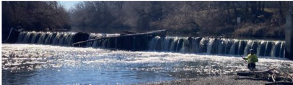
Figure 1. Low-head dam in Taylorsville
