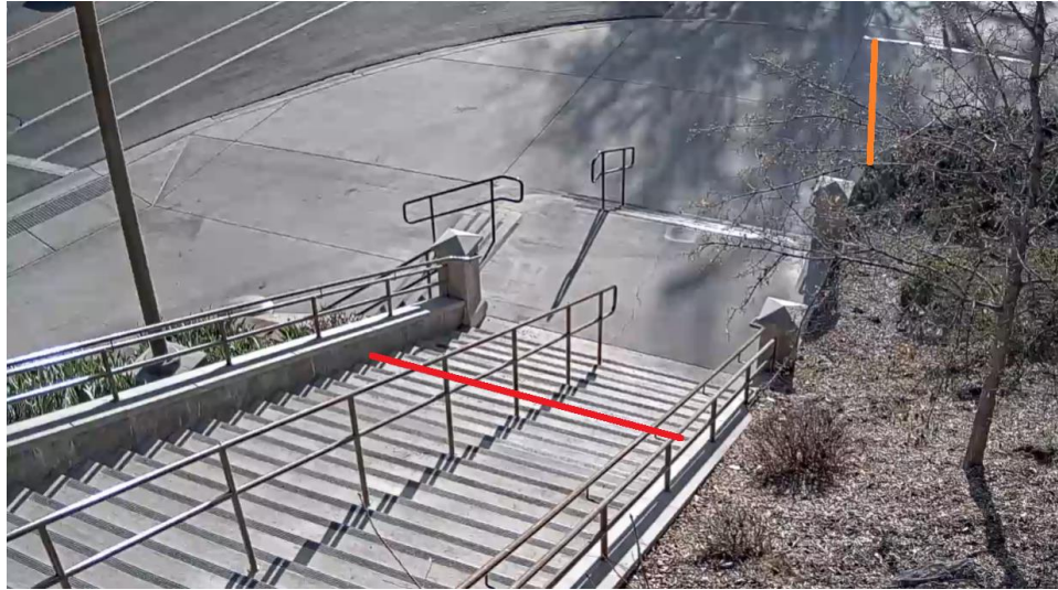
Figure 6: Approaches for the Maeser Hill Southwest Stairs location
