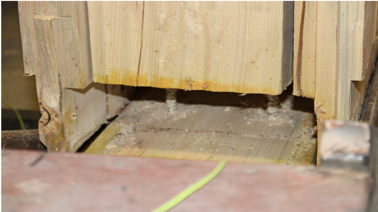
Figure 4: Wall Test 1 Pull-Out
