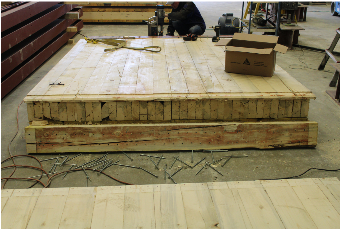
Figure 2A: Connection Screws After First Wall Failure and Disassembly
