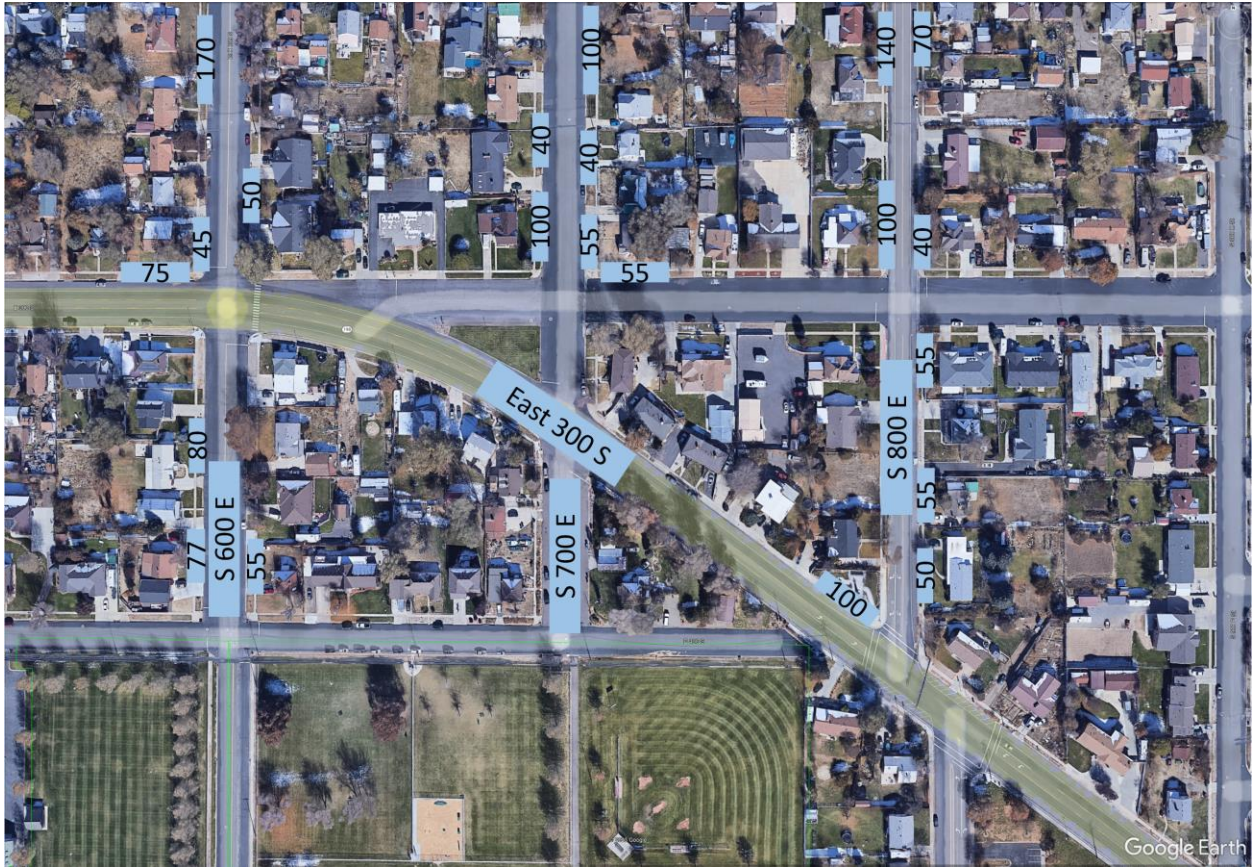
Figure 13: Tank Locations East 300 S 800 E through S 600 E
