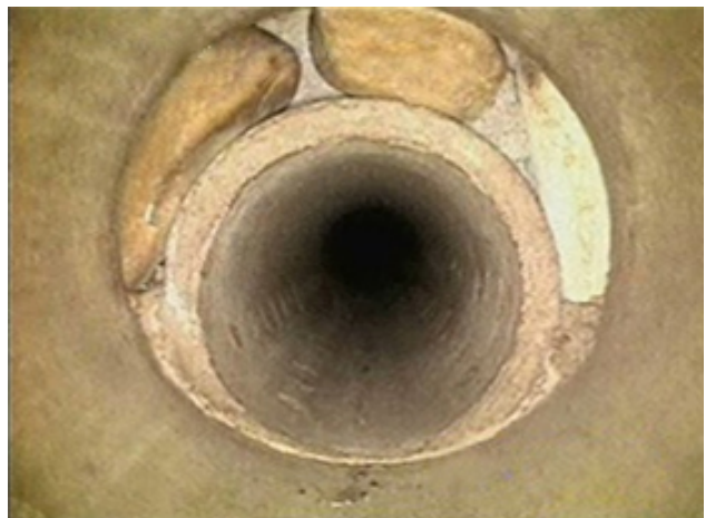
Photo 27 – View of an eccentrically constructed transition.
