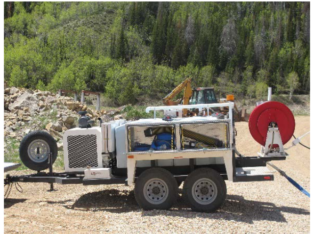
Photo 2 – View of a jetting unit used for toe drain cleanings.
