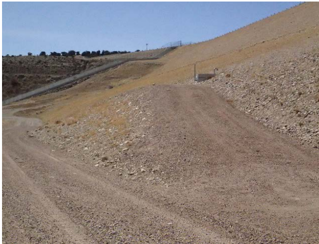
Photo 58 – View of an access ramp to a toe drain inspection well.
