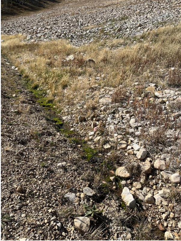
Figure 3: Significant growth on right side of dam face
