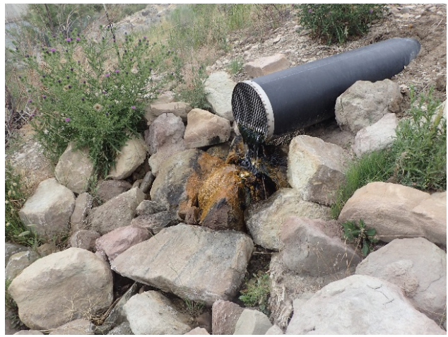
Photo 63 – View of toe drain outfall screen.
