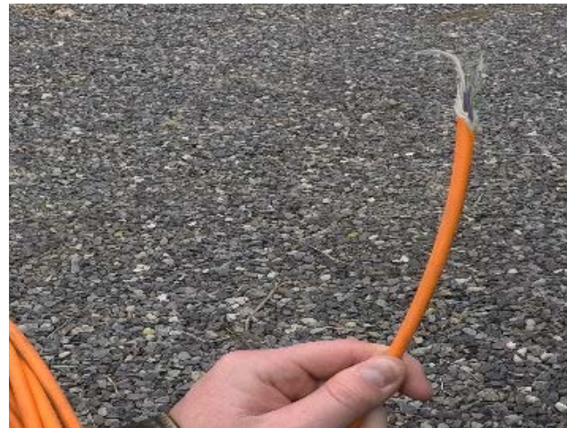
Photo 33 – A damaged CCTV cable caused by too much friction.
