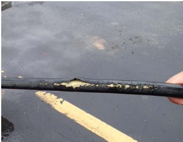
Photo 32 – Damaged cleaning hose from going around a sharp 90° elbow.
