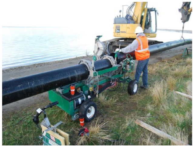
Photo 21 – View of solid walled HDPE pipe being fused at the joints.
