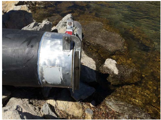
Photo 57 – View of an aluminum flap gate.
