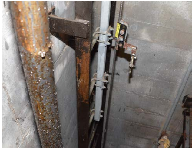
Photo 45 – View of a ladder fall protection system attached to a ladder.
