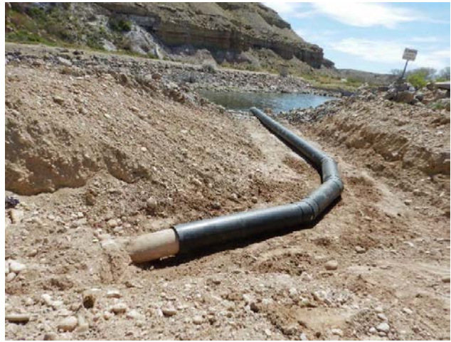
Photo 35 – New alignment of the pipe shown in Photo 34, allowing inspection access.
