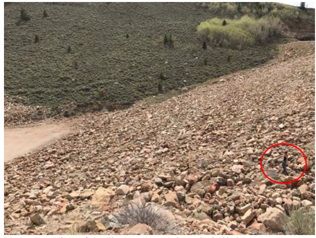
Photo 59 – View of the distance (approximately 350') between an access manhole (with a person standing on top of the cover and circled), and the trailer access road below. The distance and terrain that must be covered by the equipment prior to getting into the inspection well creates friction and limits the inspection capabilities.
