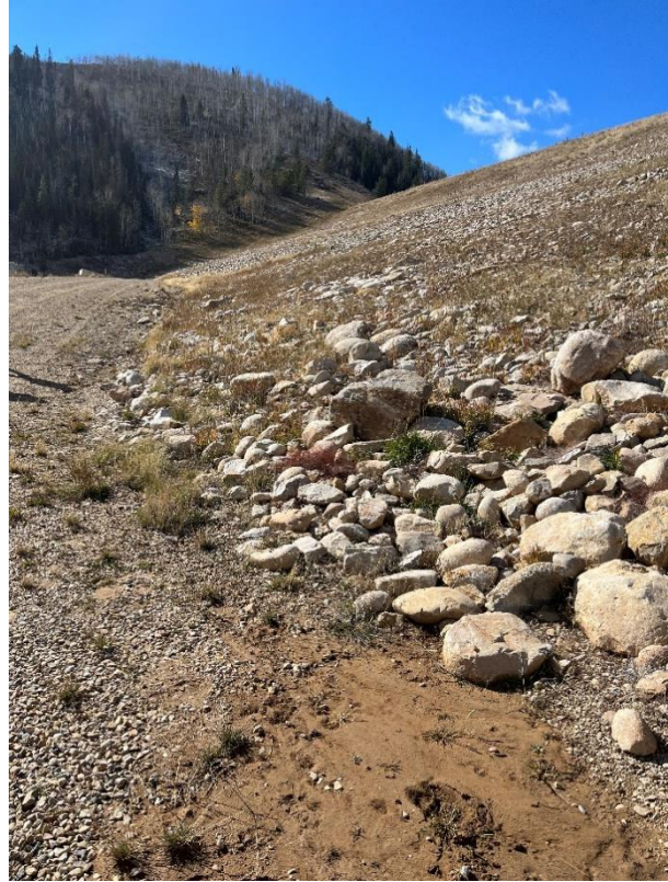
Figure 3: Significant growth on right side of dam face
