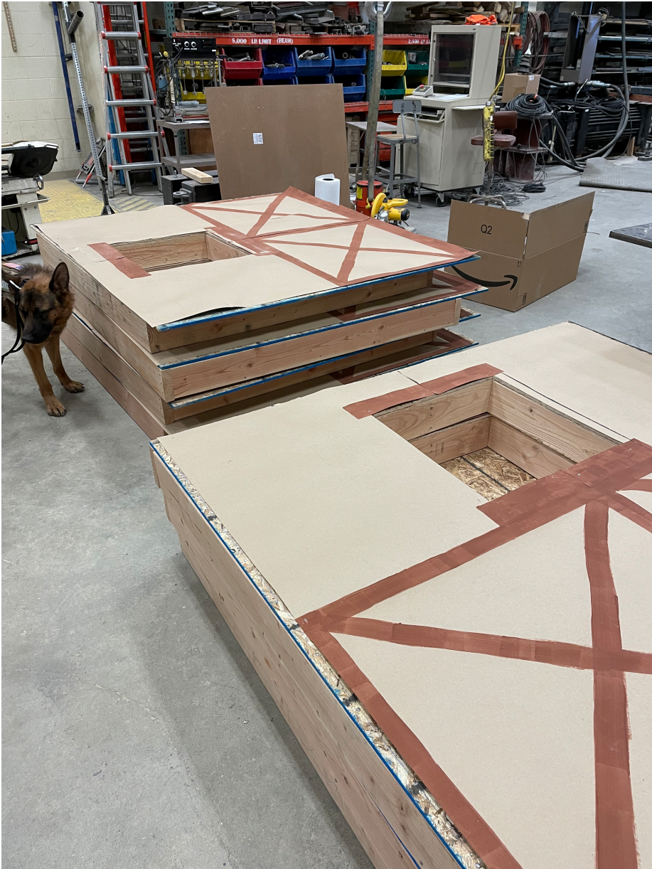
Figure 9 Decorative cardboard panels were attached to the sheathed walls.
