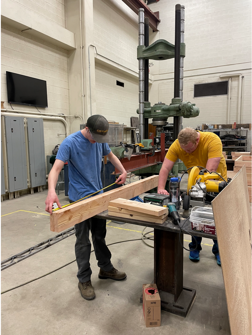
Figure 6 Team members measuring lumber in preparation to cut it for framing.
