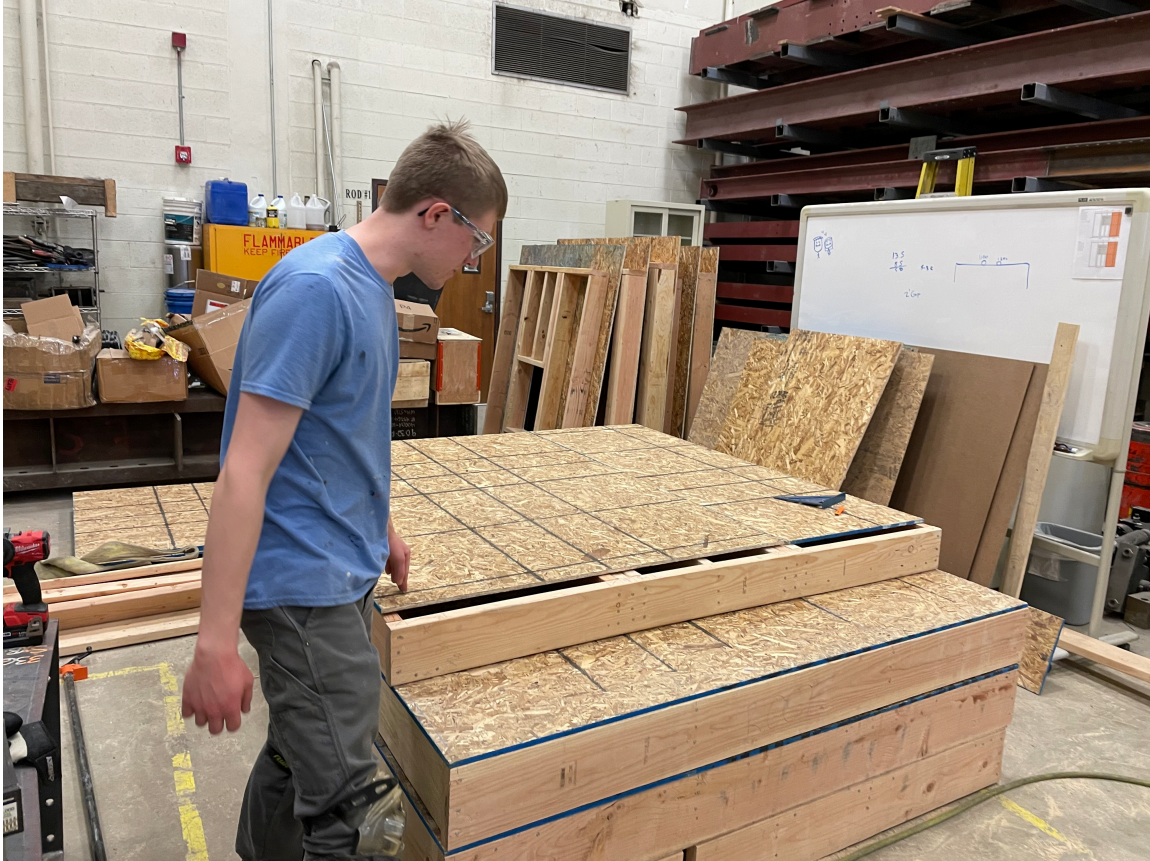
Figure 8 Our framing expert prepares to sheath a wall.
