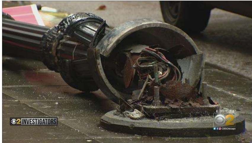
Figure 2: Damaged Light Pole in Chicago (Rusty, 2019)
