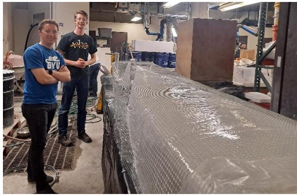
Figure 3: Steel Reinforcement Shaping
